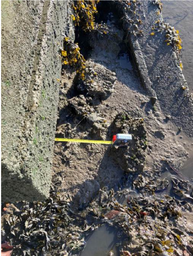
Monitoring the undercut
