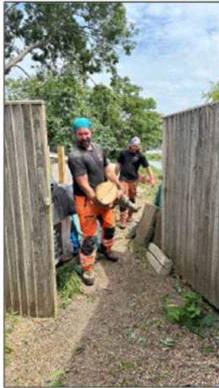
Removing the tree trunks
