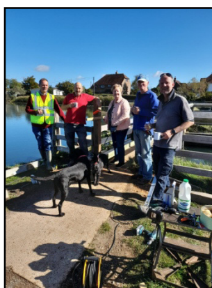
The team working on the footbridge upright posts
