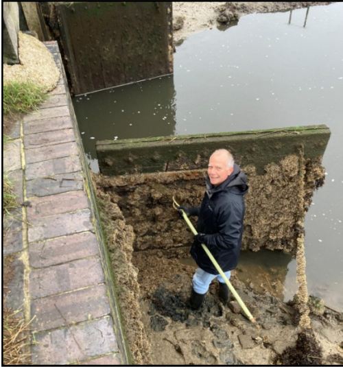
Before cleaning - Fraser Dibden showing the amount of growth on the gates
