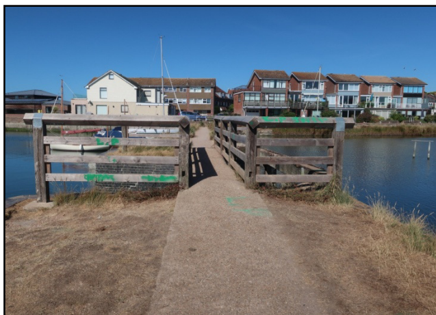
Graffiti on the footbridge – August 2022
