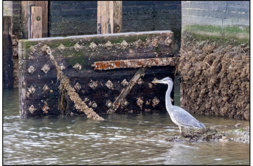
Afterwards - a heron admiring the newly cleaned gates
