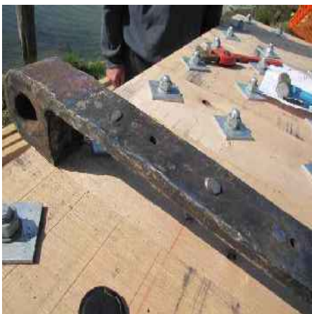
Recycled hinge being refitted
