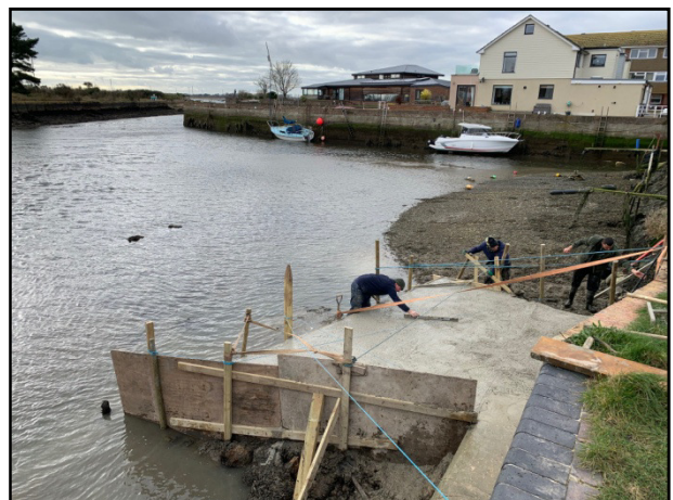
NEARLY COMPLETE – Repaired Sluice Apron viewed from footbridge
