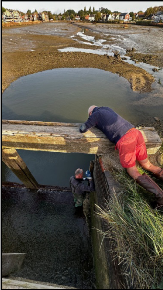
Applying the “waterfall foam” to reduce tidal gate leakage
