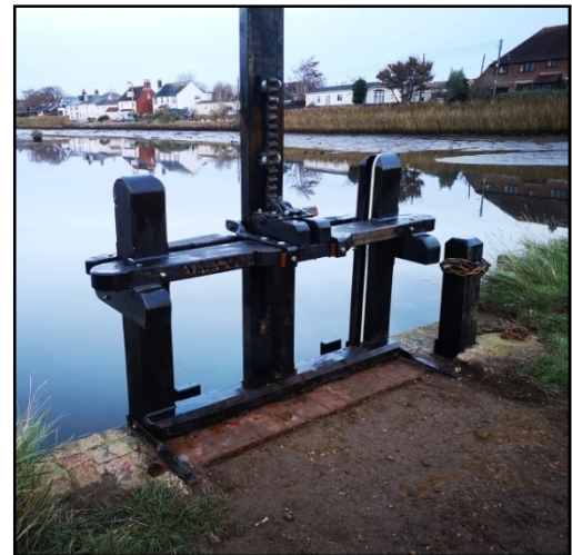
Sluice Gate after servicing by Nick Gates – November 2023
