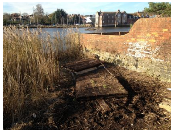
Assembly Area - note soft ground
