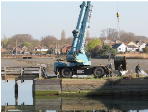
Old gates being lifted out - April 2012
