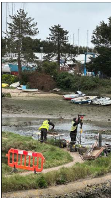
Exploratory drilling of the SW corner
