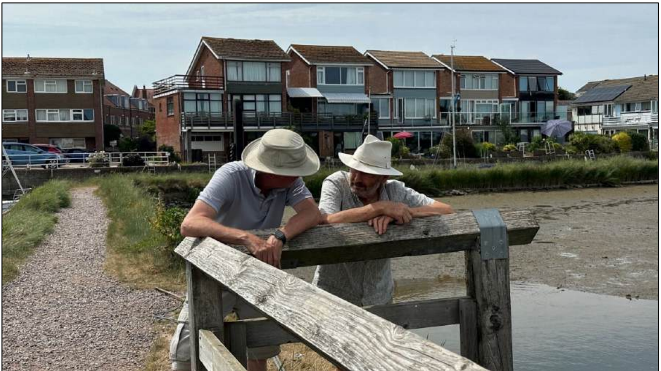
Simon Eveleigh & Nick Yoward discussing how to repair the footbridge after it had been vandalised – thankyou both!
