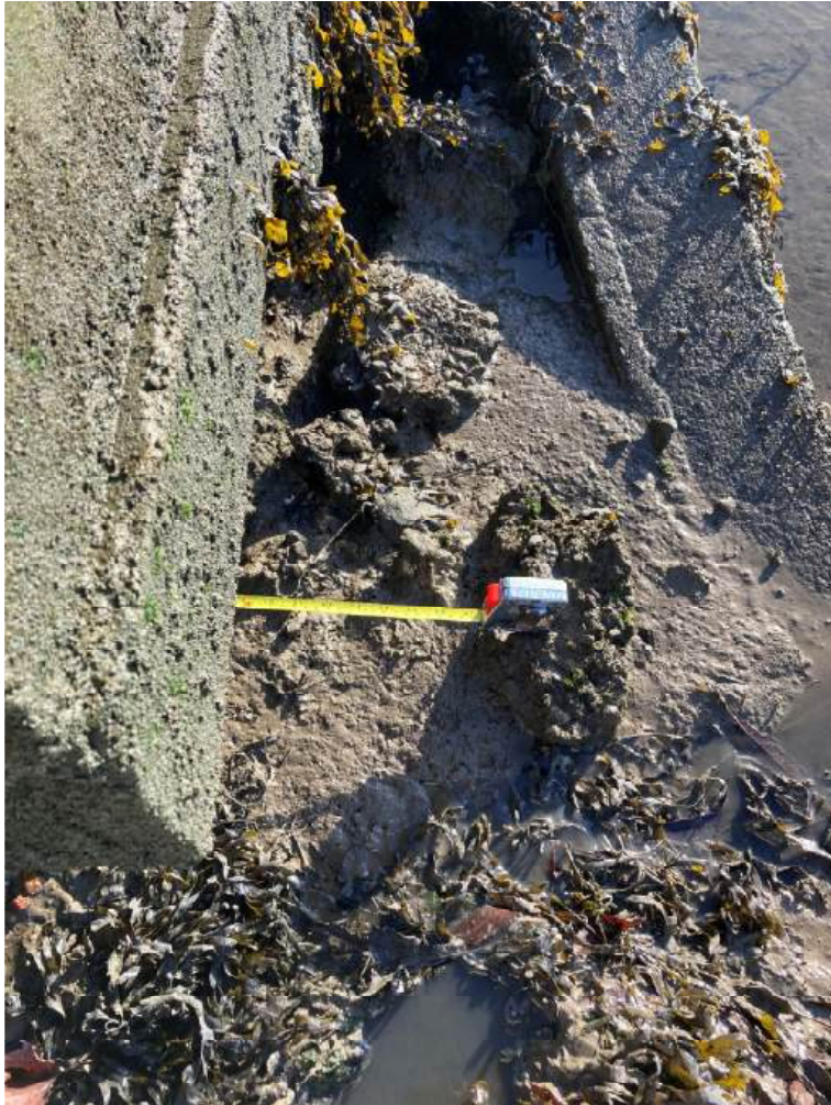
Monitoring the undercut
