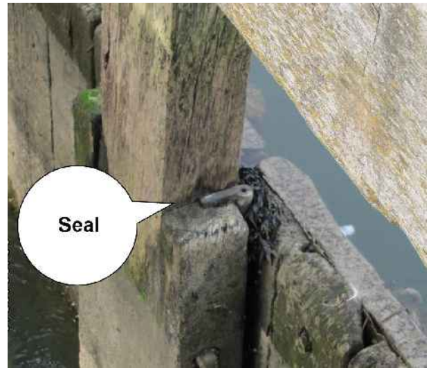
Central Post Seal Detail
