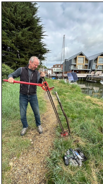
Simon Eveleigh removing a post using a farm jack
