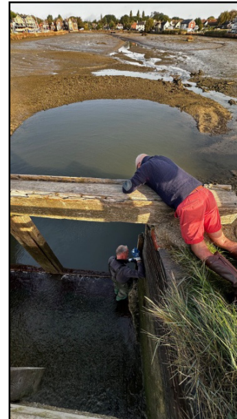
October 2023 Filling the leaks with “waterfall foam”
