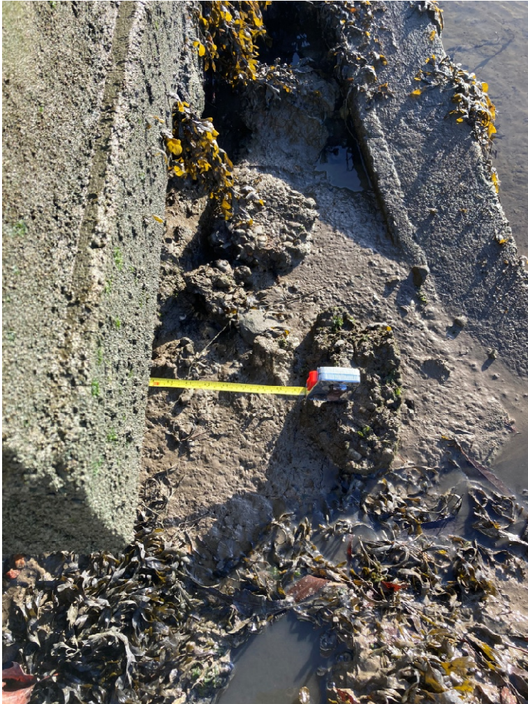
Monitoring the undercut
