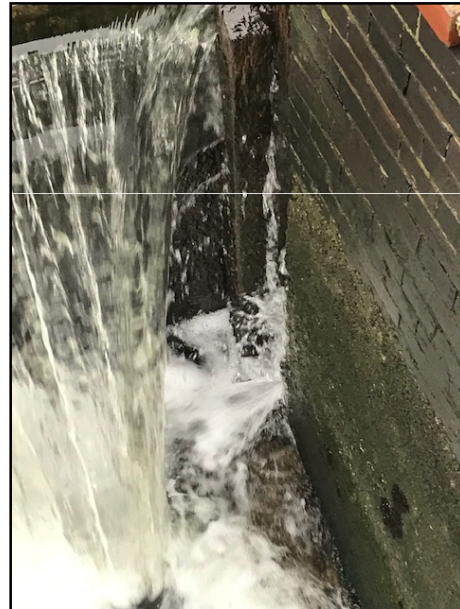
Leakage around tidal gate corner posts next to wall
