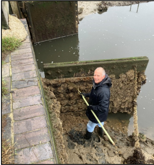
October 2022 - Before cleaning - Fraser Dibden showing the amount of growth on the gates
