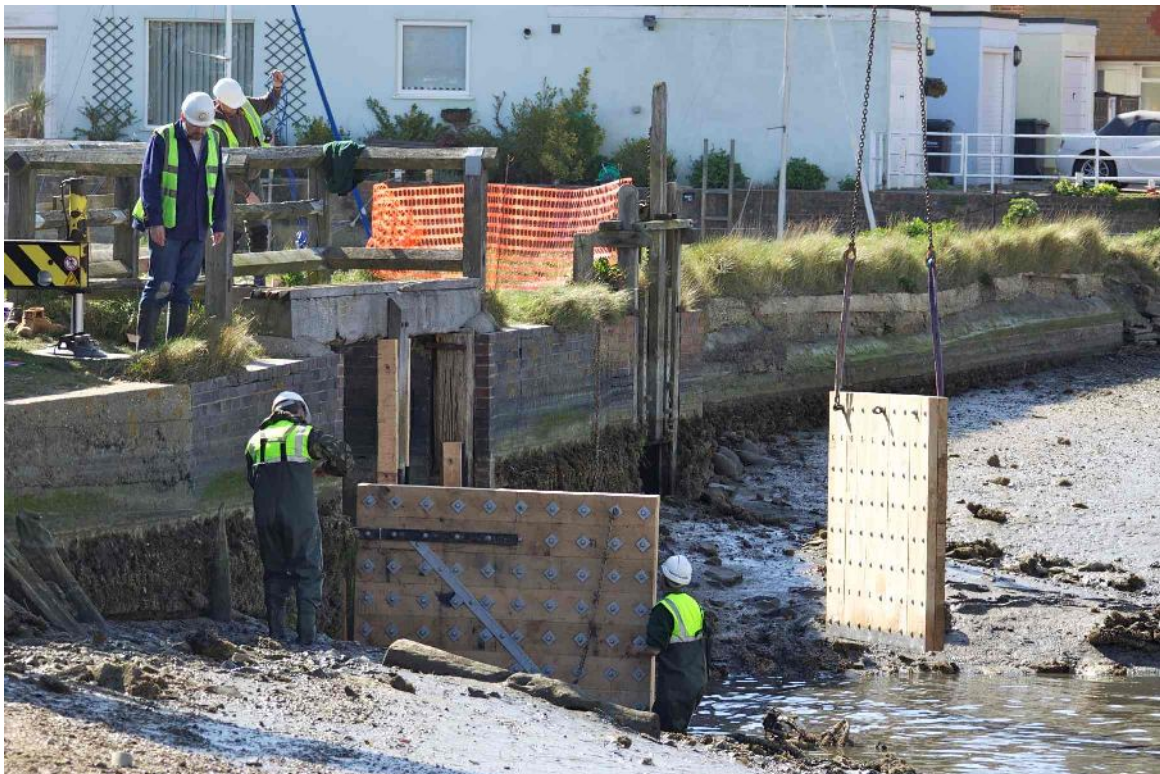
Gates being positioned
